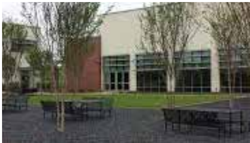
FFE Service center
